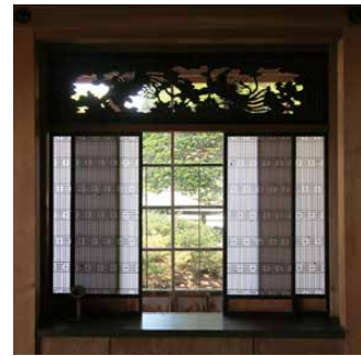
Tsukeshoin This feature, typically located next to the tokonoma , provides light for the room. The wooden ranma , a decorative transom, has some of phoenixes. The paper screen, also hand-made, has a fine wooden frame.
